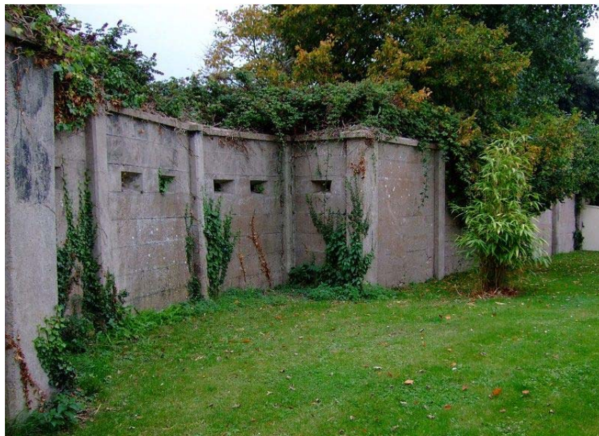
The ferro-concrete wall (thanks to Debs at http://www.fortsandbatteries.co.uk/ )
